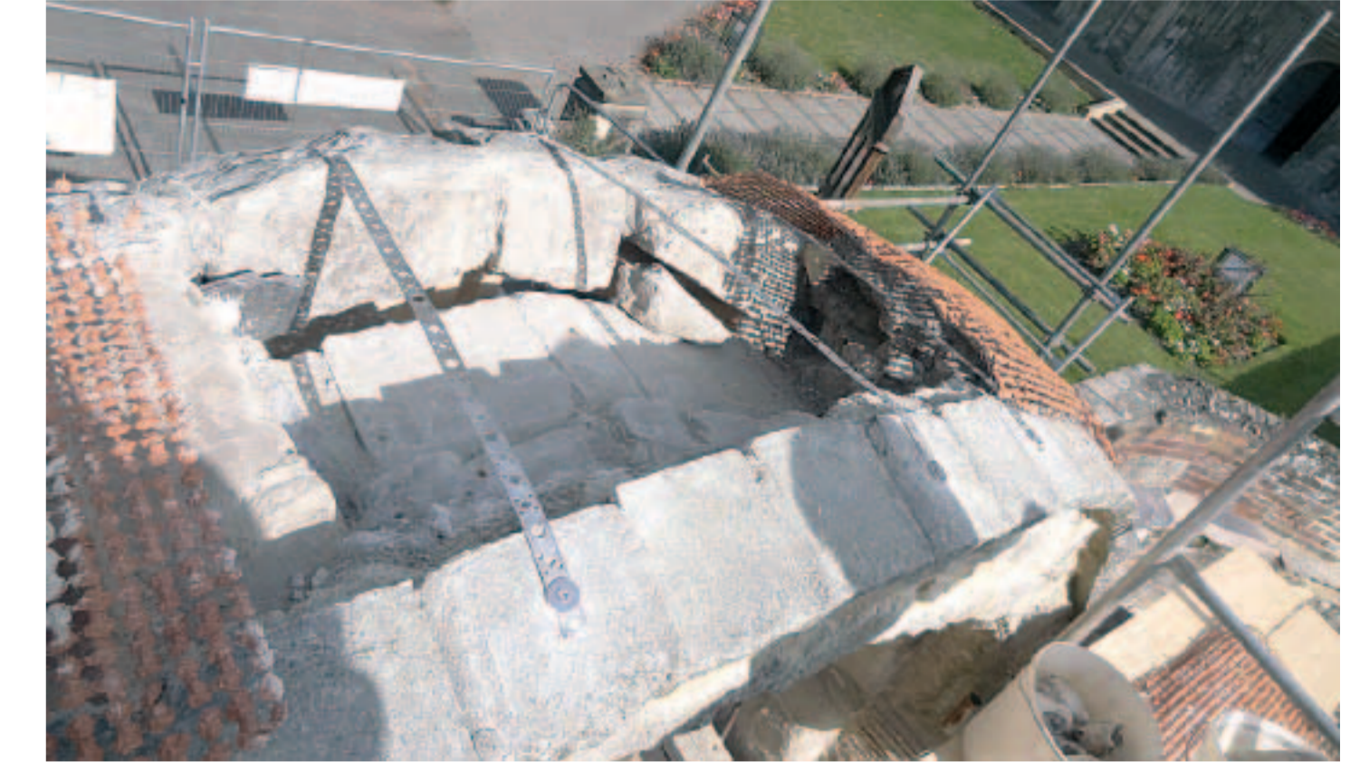
The stone arch with reinforcement
