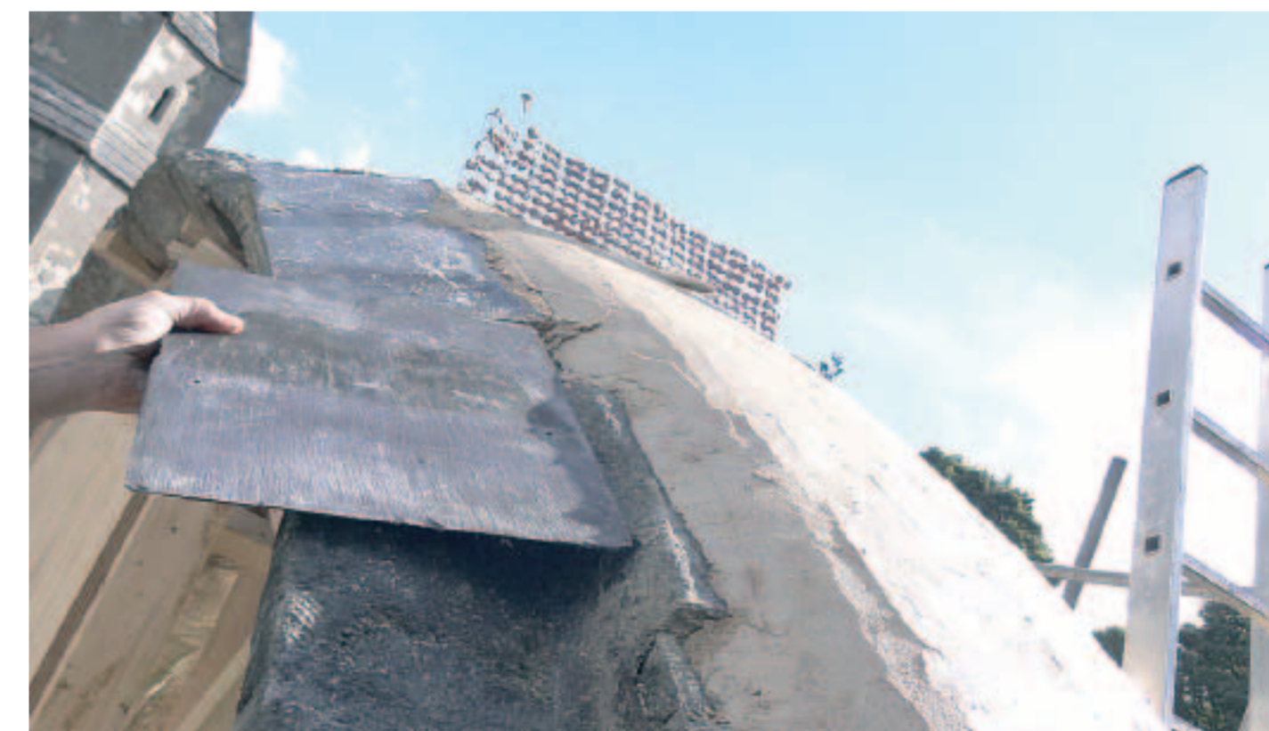
The slate was used to 'weather' the joints of the arch stones
